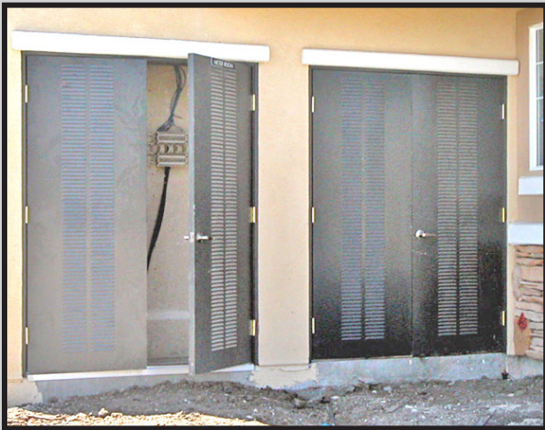
RECOMENDED - The mechanical and electrical equipment for this building has been successfully concealed within the building with louvered doors and trim painted to match other elements on the building facade.
