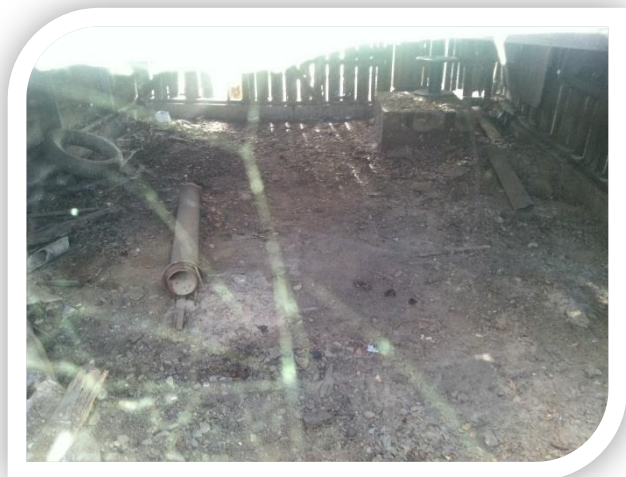
Above: Inside the small wooden barn. At the time of our visual inspection, pipes, wood and tires appear to be the only materials stored in the structure.
