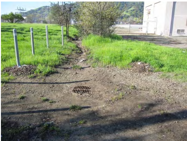
Photograph 3. Drainage ditch leading from the secondary containment basin to a storm drain, looking west.
