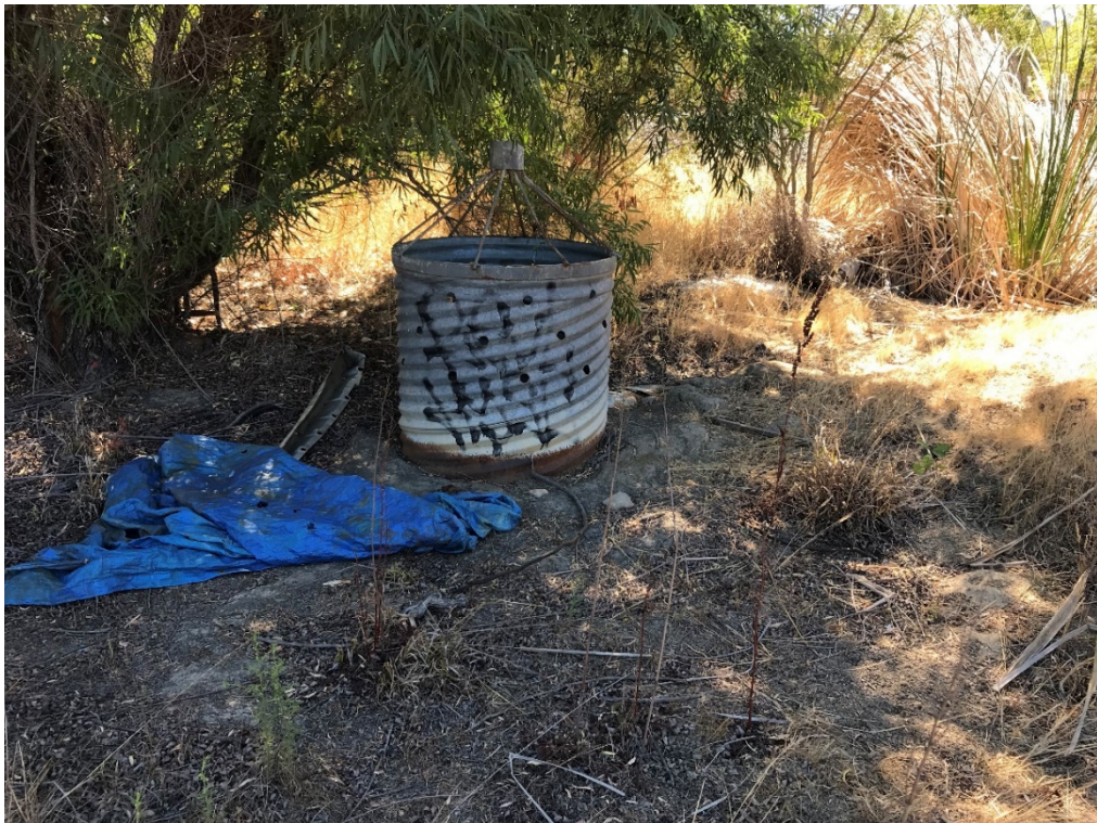
Photo 10. Standpipe in detention basin
