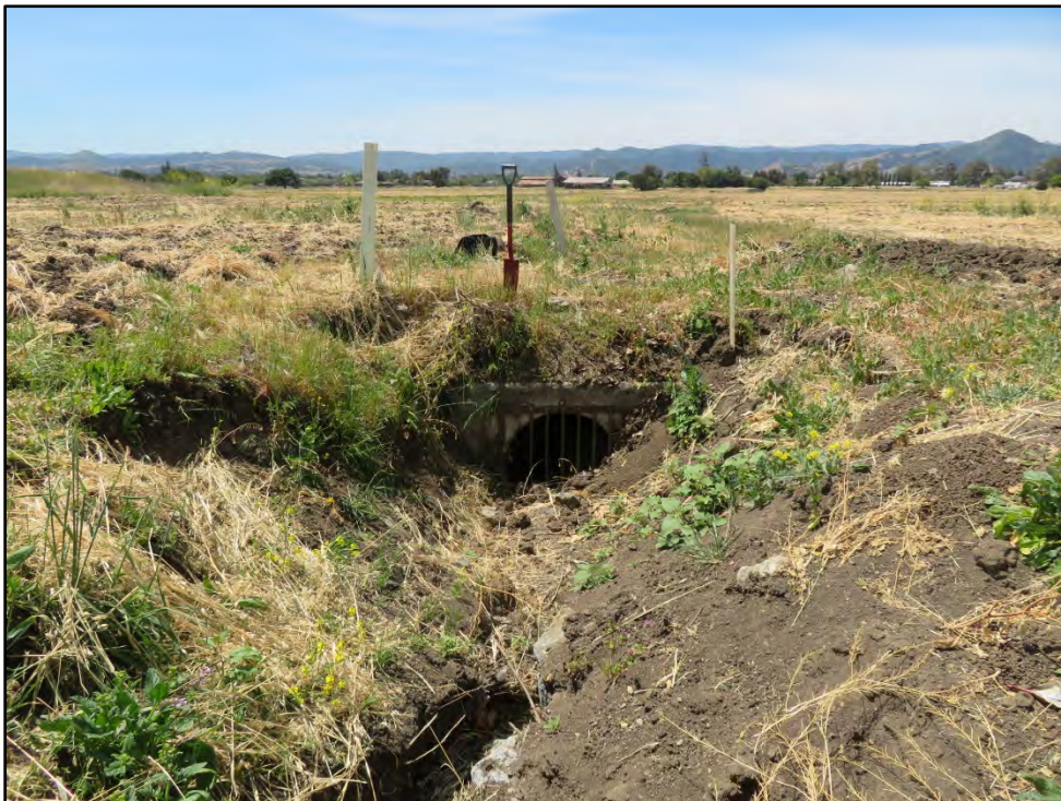
Photo 10. Storm drain culvert at the downstream end of the ephemeral drainage.
