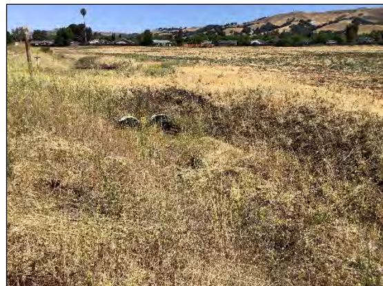
Photo 6. Culvert in Tennant Creek to be removed and the banks graded to match the adjacent slopes.
