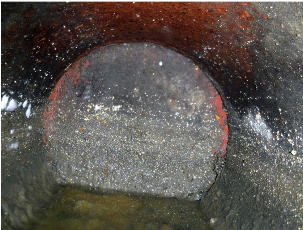
Photo 2-4. Manhole G4-D.MH.040 SE Effluent Line (Capped)
