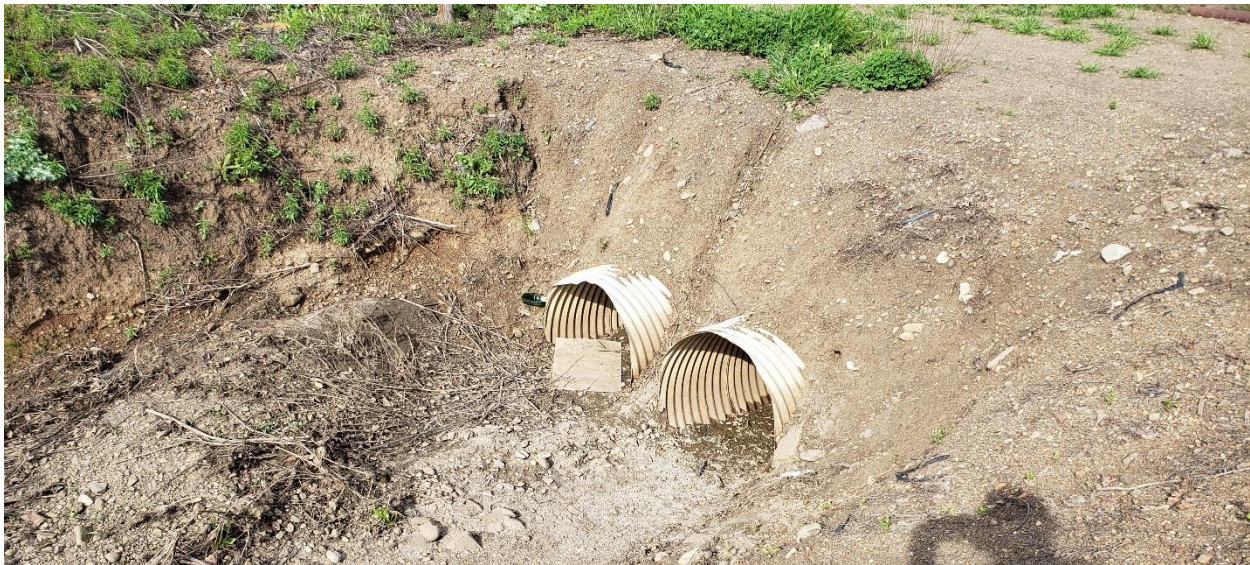
Figure 3-1: Existing Twin 36-inch CMP Culverts on the Project Site
