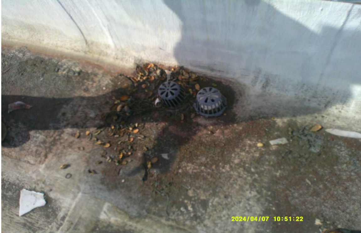
Overview of sumped internal drain and overflow.
