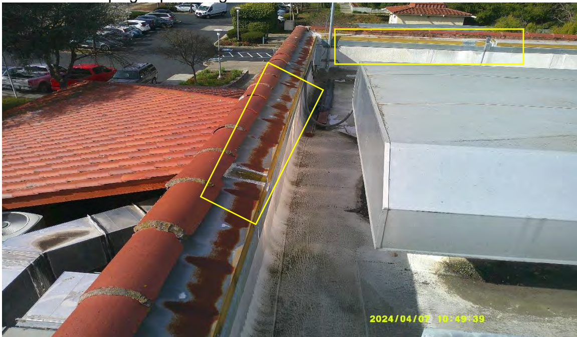
Overview of coping cap and reglet detail.
