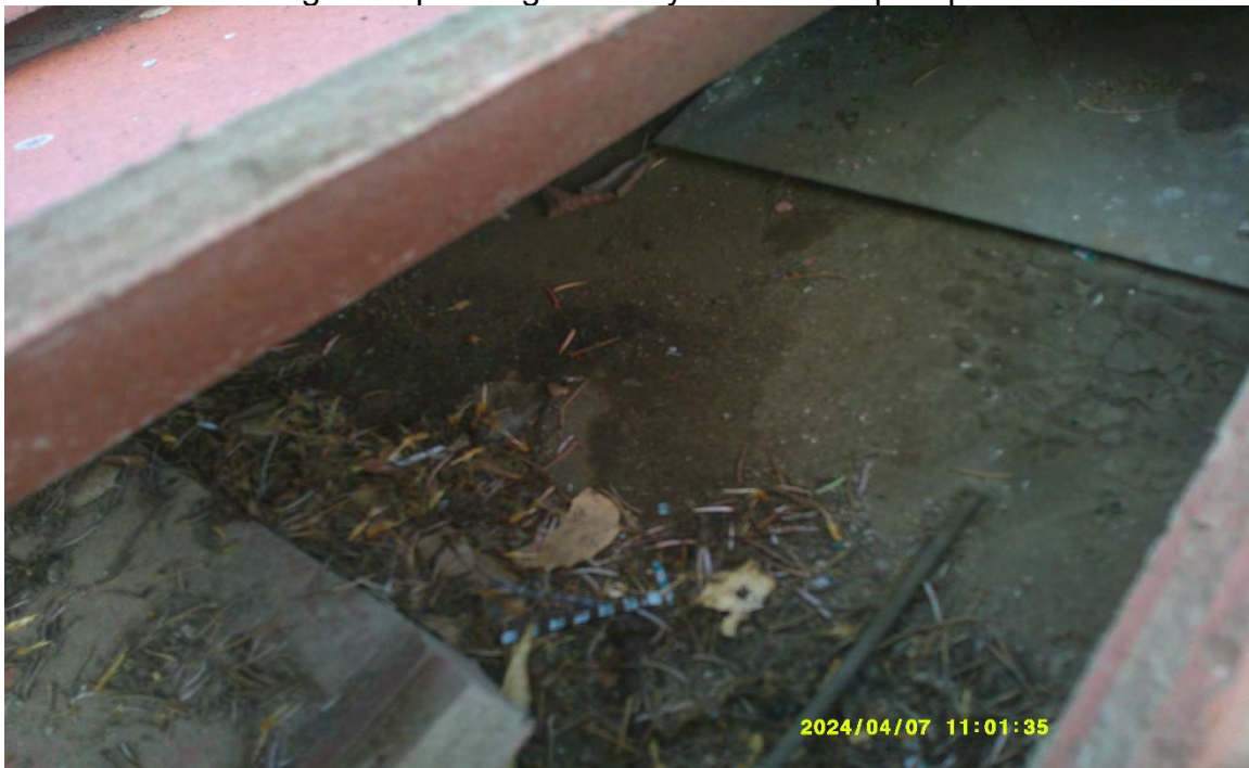
View of deteriorating waterproofing underlayment at steep sloped roof area.
