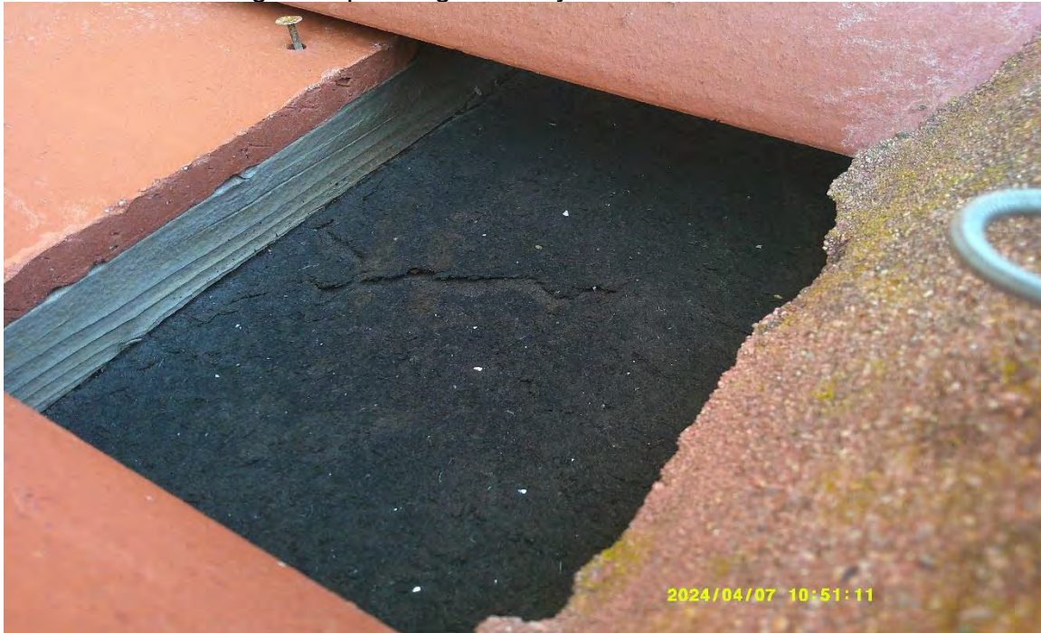
View of deteriorating waterproofing underlayment at mansard.
