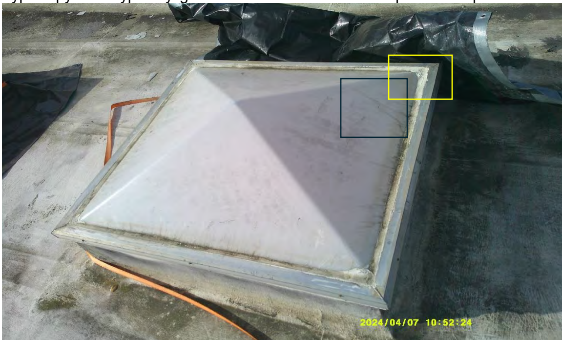
Typical pyramid type skylight condition notes cracks and previous repairs.
