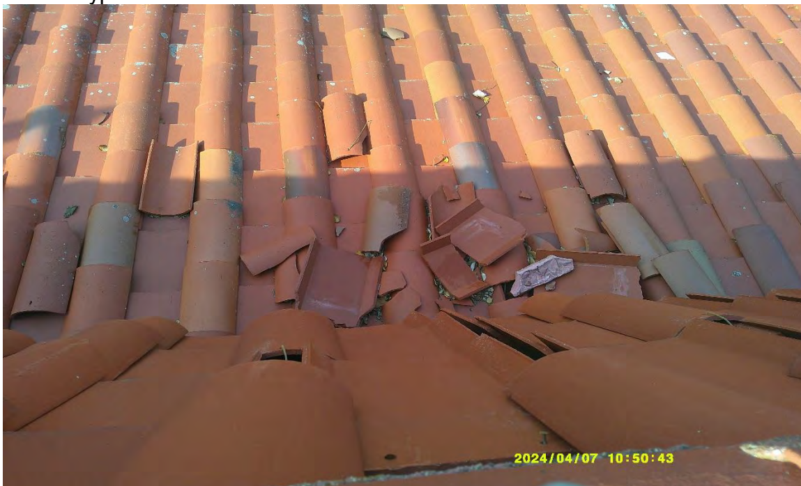
View of typical broken tile.
