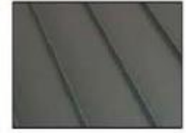
Standing Seam Metal Roofing
