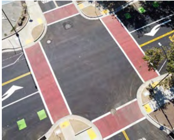
FIGURE 45 Curb extensions (Source: Caltrans)
