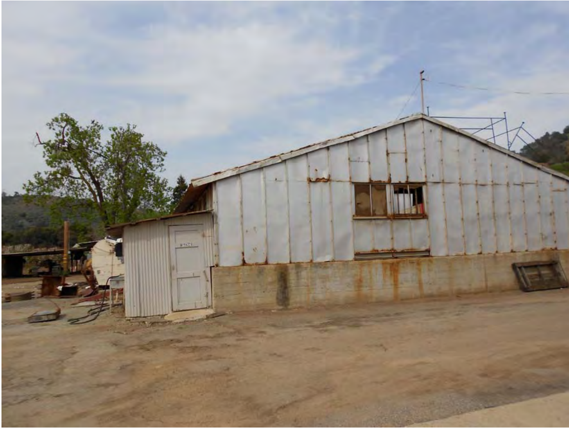
Photograph # 10 The south facade of the “sulfur” house showing the raised seam metal siding, small metal frame windows, and concrete base wall. The building is in fair to poor condition with deteriorated metal siding that is pulling away and rusted. Windows that are broken and patched with miscellaneous materials.
