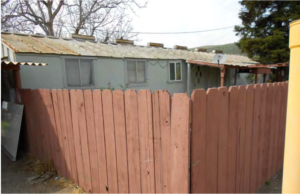
Photograph # 7 Residential building of mixed materials. Wood panels cover the front and raised seam metal siding is on the ends. The roof is "button" raised seam sheets of galvanized metal. The building was moved to the property in the 1950's..
