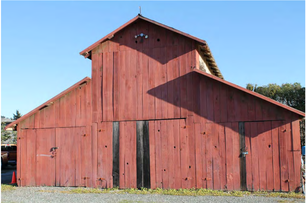
Barn c.1935 The barn is a remnant of the previous farm/ranch use and is currently used for miscellaneous and vehicle storage. The vertical board construction is typical for ranch barns of the 1900-1940.
