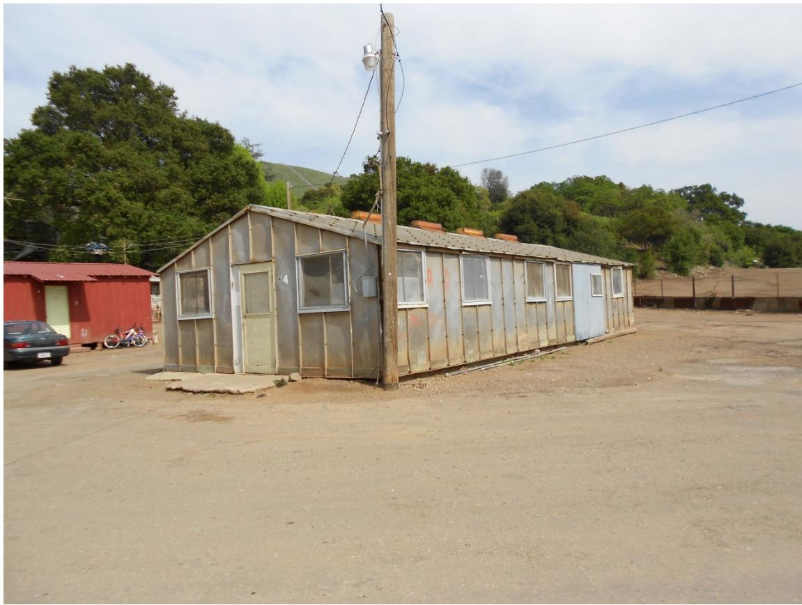
**Photograph #4 Worker's housing; metal frame, "button" raised seam metal siding.**
