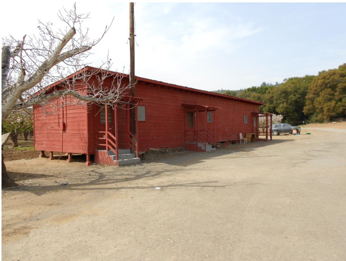
**Photograph # 2 Multiple unit ranch worker housing. The building is wood frame with horizontal siding. According to Chris Borello, this building was moved to the property in the 1950's. The original location is unknown.**
