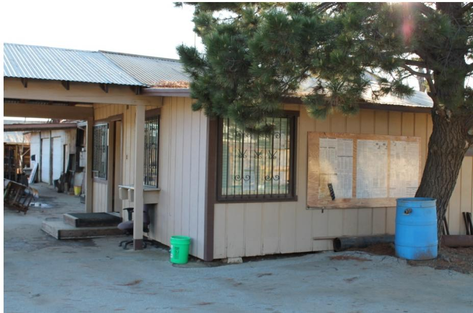
**Photograph # 12 Side of the office building, concrete pier foundation and pitched roof. The windows are covered with decorative security grills. The building is a modular building, c.1985**
